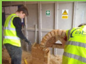
Here Alfie and TJ used a semi-circular timber turning piece to form the arch.
