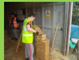
The brickwork was half round jointed by TJ and Alfie and the work area is cleaned and tools tidied away. Both work safely attired in the correct Personal Protective Work wear and followed a safe system of work.
