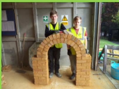
Alfie is laying the second ring of bricks to form the arch
